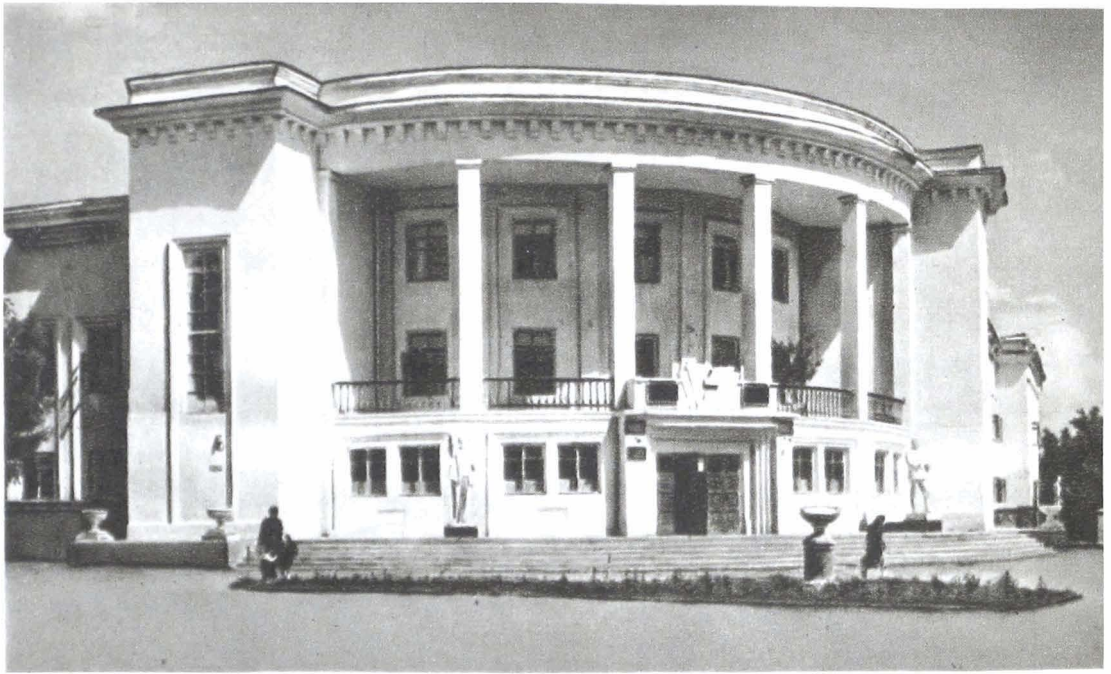
The Central Polyclinic in Krasny Partisan Street, Stalinabad
