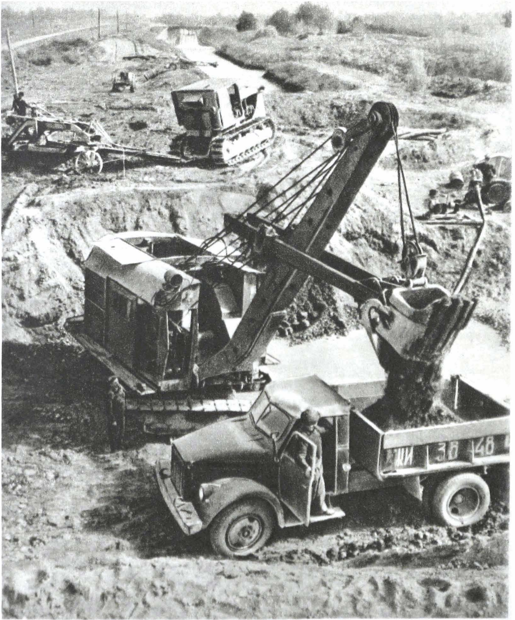
Irrigation work in the Vakhsh Valley. Digging canals in the Kurgan-Tyube District
